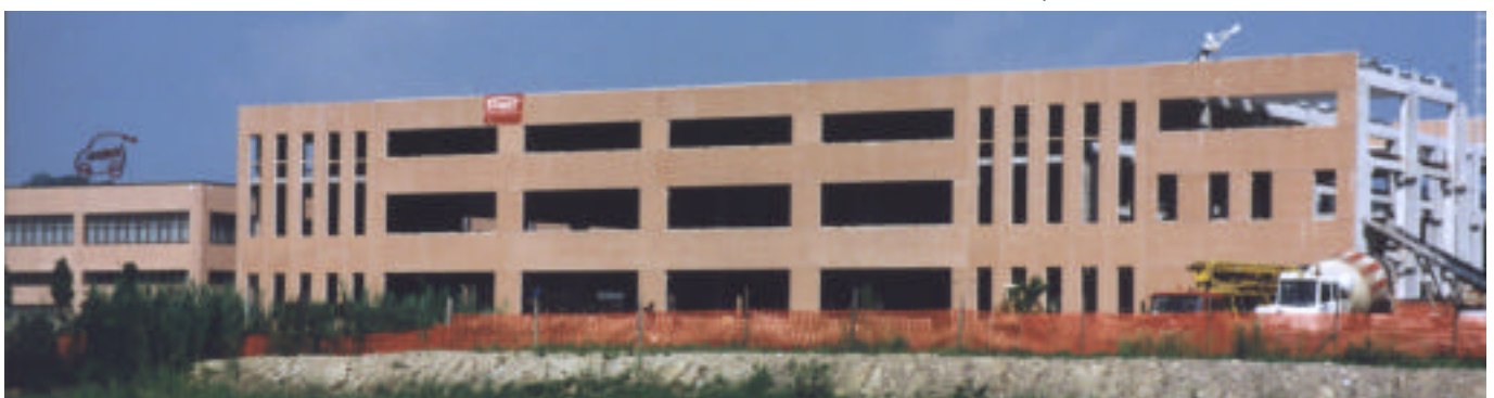
Figure 6. ZEBRA battery production plant (Phase I) under construction
